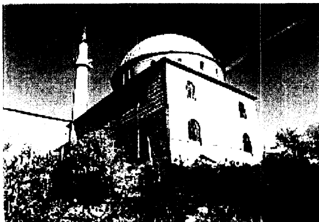
pre-war photo from: Raif Virmica - view from SW with minaret
