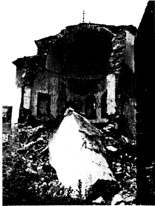
photo by: Sabri Bajgora (1999) - view from rear, showing collapsed rear wall, burned-out interior
