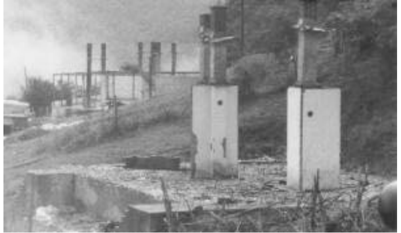
Destroyed school in Kotlina [zoom]
