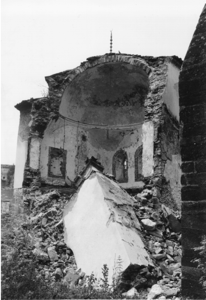
Figure 7. Gjakova/Djakovica (Kosovo). Library of the Mosque of Hadum Suleiman Aga, founded in 1595. The library was burned by Serb troops at the end of March 1999. Its rear wall was smashed in May 1999, when the top of the minaret of the adjacent mosque was shot off and toppled onto the library building. (Photo courtesy of Prof. Sabri Bajgora, Faculty of Islamic Studies in Prishtina.)
