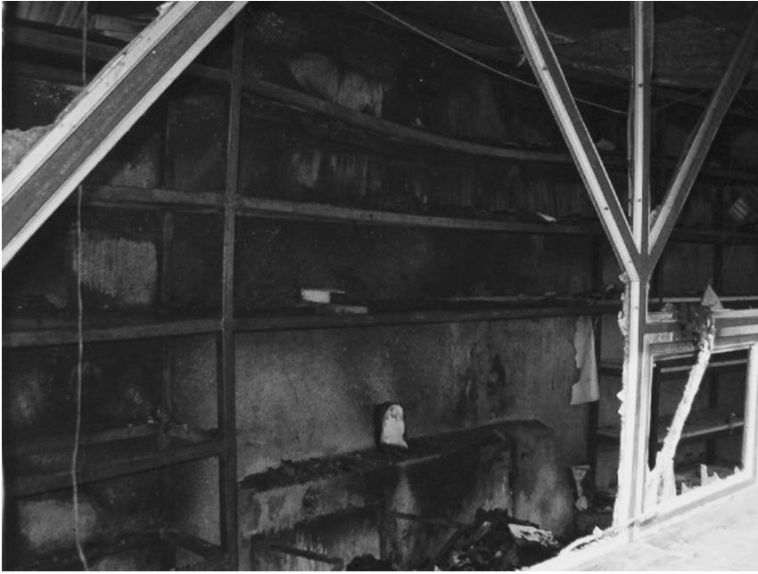
Figure 8. Belgrade, Serbia. Library and archive of the Islamic community of Belgrade, sacked and burned by a mob, March 18, 2004. (Photo courtesy of the Islamic community of Belgrade.)
